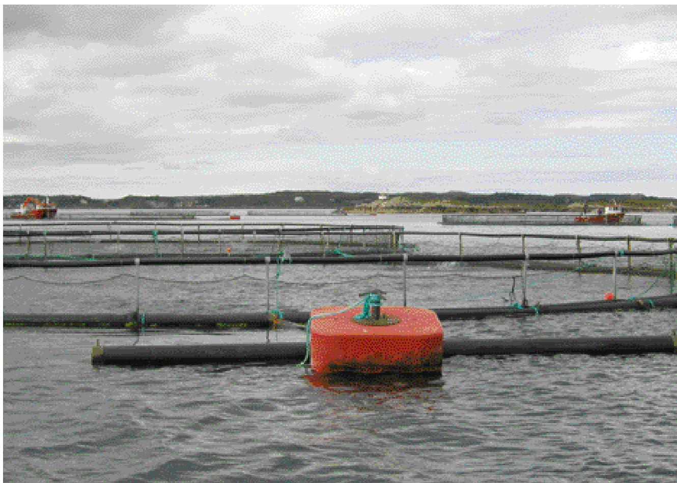
Fig 6.7 Pairs of circular collar cages attached to single point moorings (SPM's). Aqualine, Norway.
