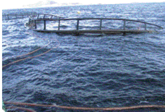
Fig 4.17 Polarcirkel cage being submerged. Polarcirkel, Norway.
