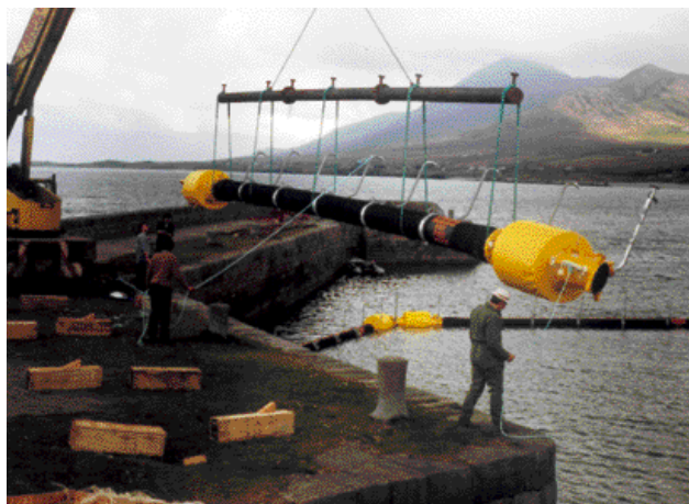
Fig 4.6 Crane lowering rubber pipe section for assembly of Bridgestone cage, Clew Bay, Ireland, 1987. Marine Harvest, Ireland.
