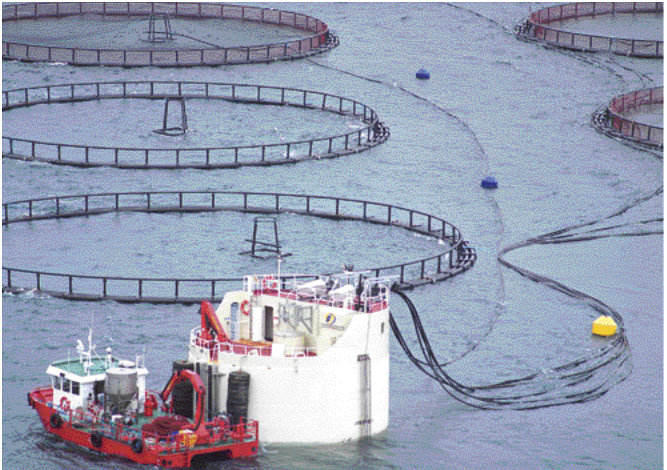
Fig 3.23 Workboat moored to concrete cylinder feed barge, Shetland Islands. Note floating feed pipe to each cage. Gael Force, Scotland.
